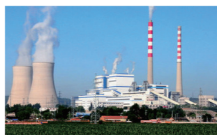
▲ 发电厂除尘 Power plant
